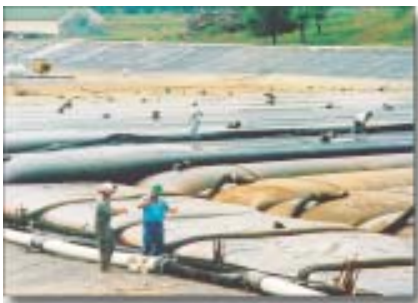
Geotubes, 20' x 200' geotextile fabric containers, were used to separate the water and sediments in the Laydown Area.
